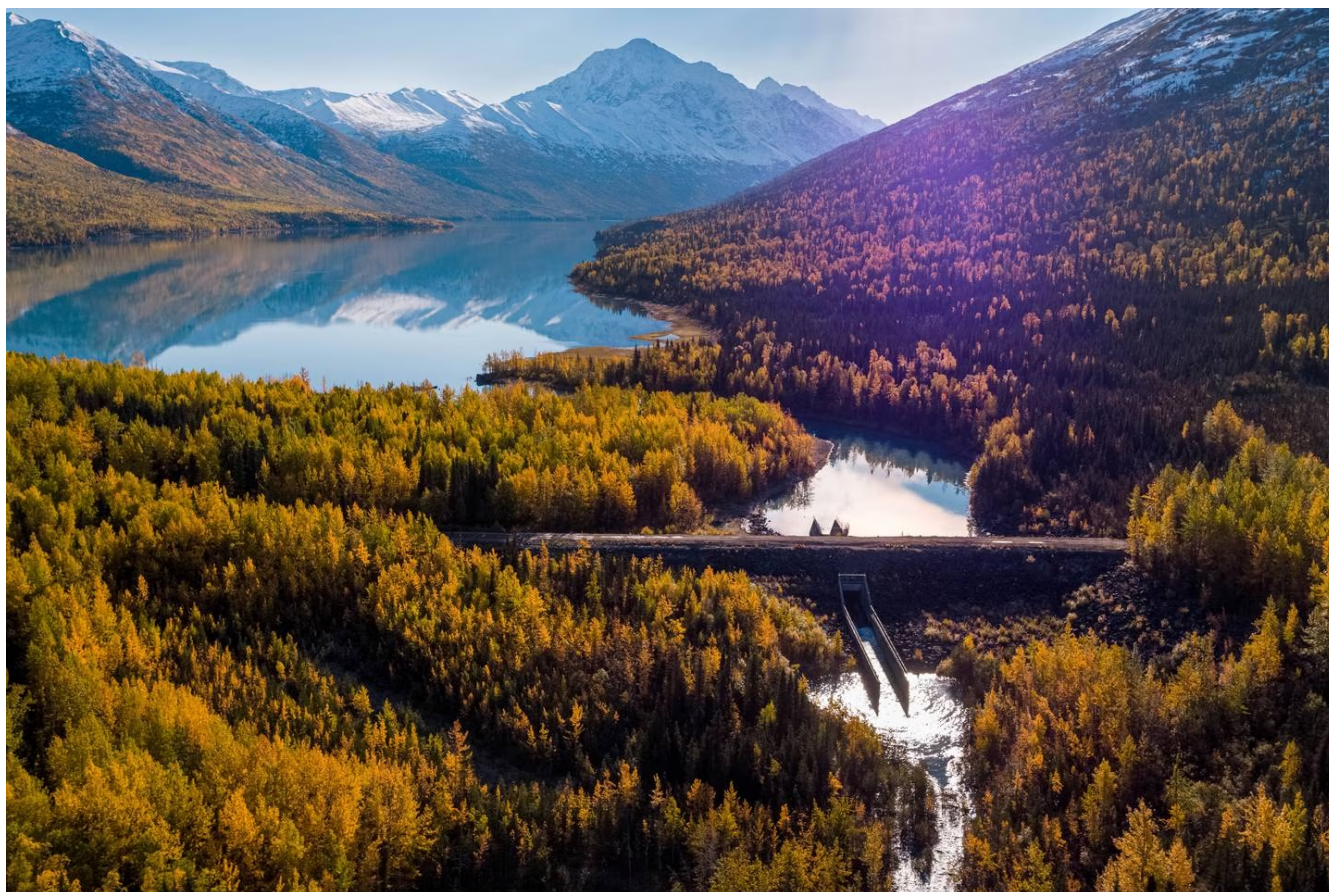
Water is released from the a dam on the upper Eklutna River on Wednesday, Sept. 22, 2021 near Eklutna Lake. The dam has been closed and the river has been dry for many years, with most of the water diverted to produce power and supply Anchorage with drinking water. (Loren Holmes / ADN)
