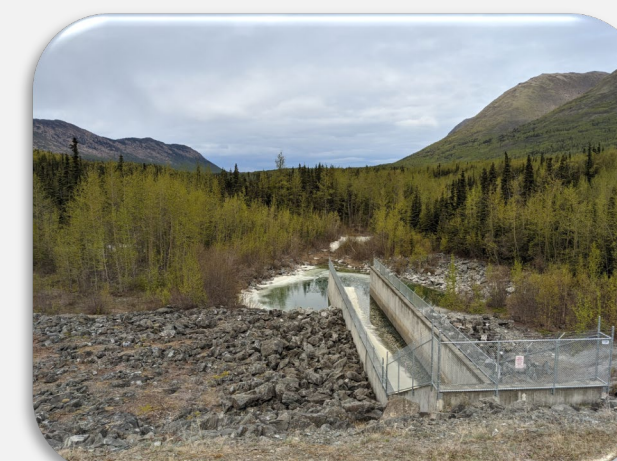
Spring photo showing no water flow through the dam .
